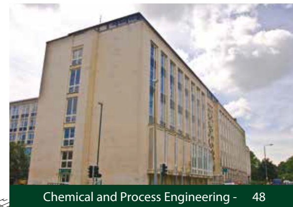
Chemical and Process Engineering - 48
